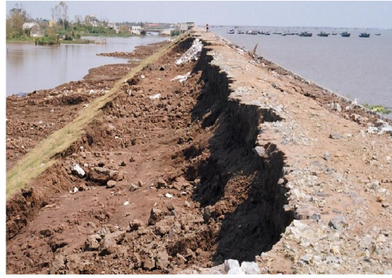
Sea dike no.3 (Tiên lãng, Hải Phòng) was broken due to typhoon no. 7/2005
