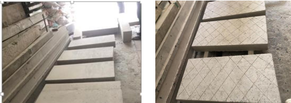
Fig. 3. Cleaning and roughening the slab surface before applying the strengthening layer.
