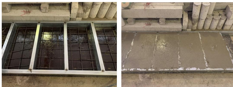
Fig. 2. Reinforcement work, formwork, and concrete pouring of the reinforced concrete slab.
