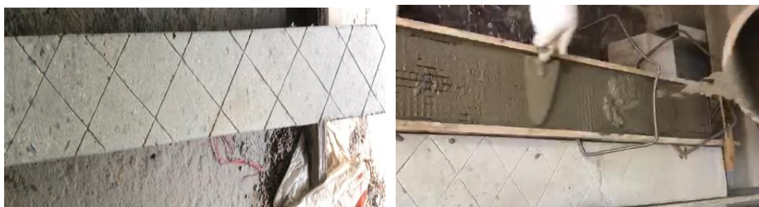
Fig. 4. Cleaning, roughening the surface, and applying the TRC layer.
