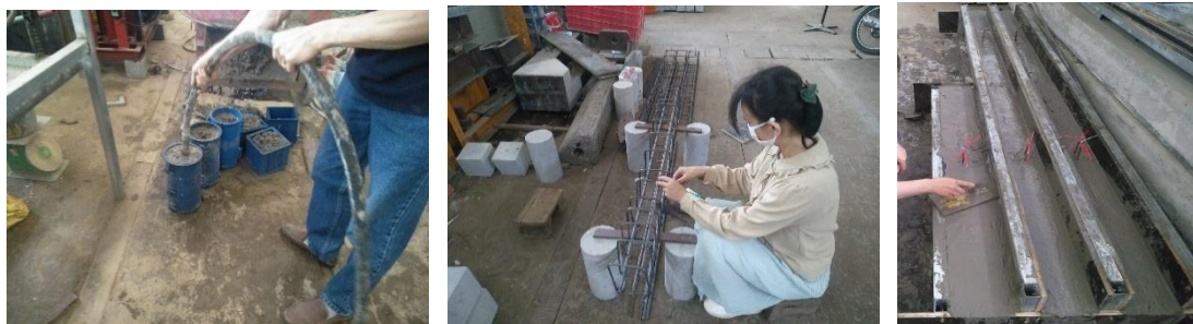
Fig. 3. Casting concrete samples, reinforcing steel, and finishing the surface of the beams.
