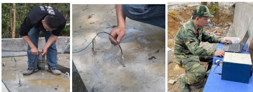
Fig. 4. Installation of water pressure sensors.
