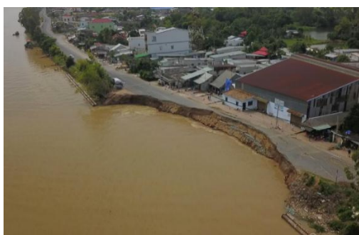
a) Riverbank erosion on Highway 91 - An Giang
