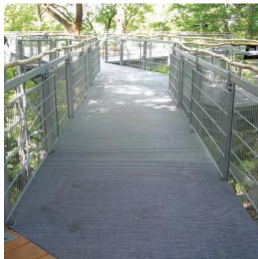
Figure 2. Joining the grating panels into the floor.
