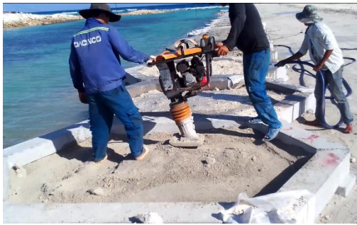
Fig. 5. Compacted coarse sand with 7% cement.
