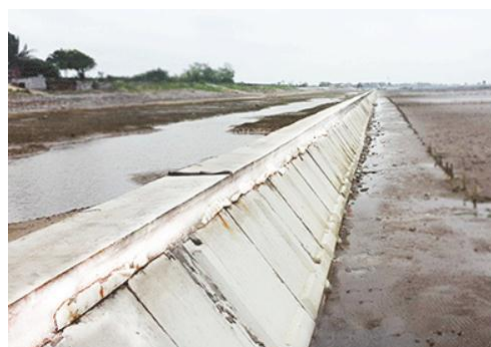
Fig. 3. Precast structures were built to prevent coastal erosion in Thai Binh.
