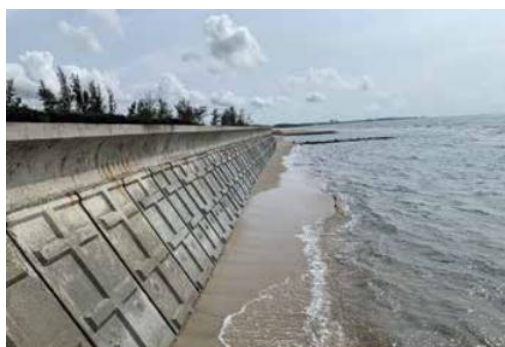
Fig. 2. Fishing Village - Xuyen Moc revetment using non-metallic reinforced concrete.
