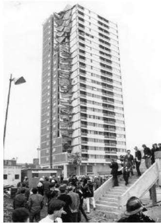
Fig. 1. Ronan Point apartment building was collapse in London in 1968.
