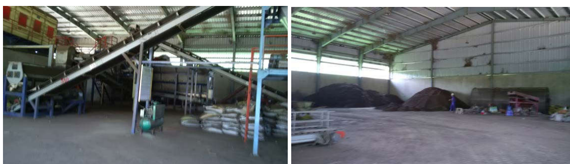
Figure 3: Lao Cai waste treatment plant
