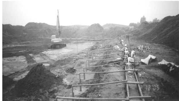
Figure 8. Hiep Thuan culvert was excavated in dry condition.
