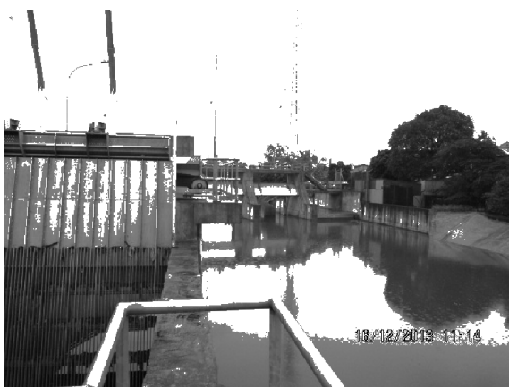
Figure 1: Typical open channel sewer system in Hanoi City close to Yen So Park WWTP
