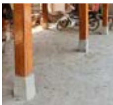
Figure 8. The details of column footing
