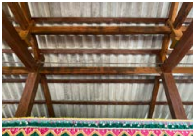
Figure 10. The structure of Column - cross beam - horizontal beam
