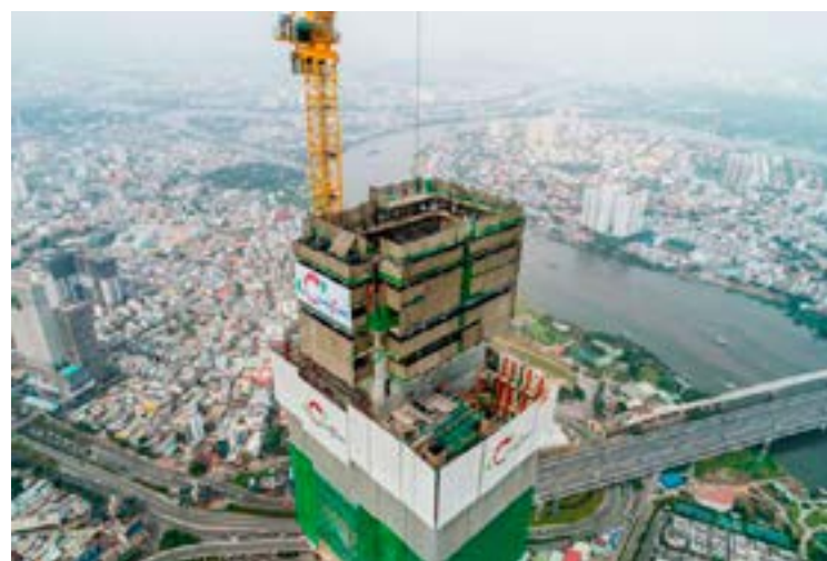
Figure 3. Climbing Formwork used at Landmark 81 project. Source: https://www.coteccons.vn
