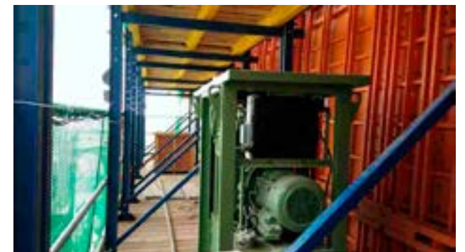
Figure 5. RCS- P (Rail Climbing System Protection Panel) used at Landmark 81 project. Source: https://coffanhom.com
