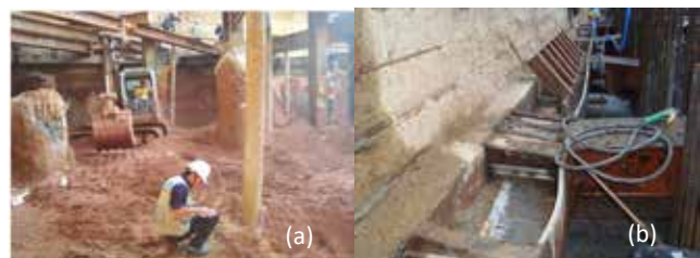
Figure 7. (a) under excavation of B3; (b) The 3 rd level of walling beam & struts status
