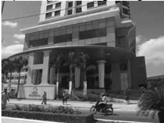
**Figure 7.** Expanding the canopy with the support structure "disguised" with a logo and a high platform that prevents visibility and communication between the building and the street space. Source: Author
