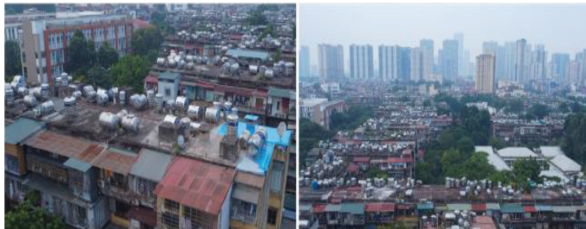
(a) Water tanks on the roof (b) Panoramic view of the city Image 1. Rooftops of old apartment buildings have become areas for water tanks, unintentionally degrading urban aesthetics. Source: Authors
