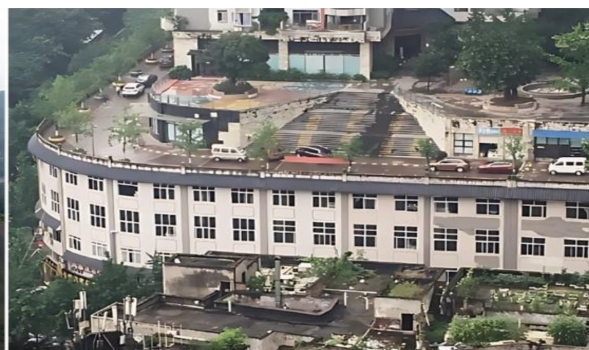
(b) Rooftop parking and roads
