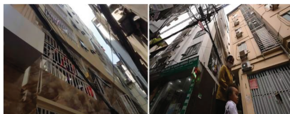
(a) Tangled electrical wire (b) Air conditioner outdoor units
