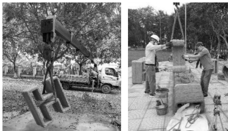
Figure 7. The process of transporting and erecting the logo
