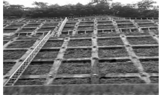
Figure 5. Hybrid crib-anchored retaining wall
