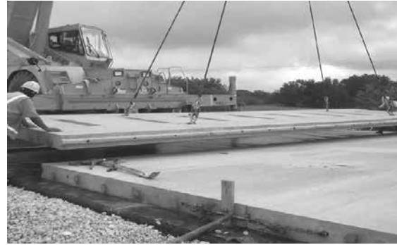
Figure 3. PPCP: Construction and installation
