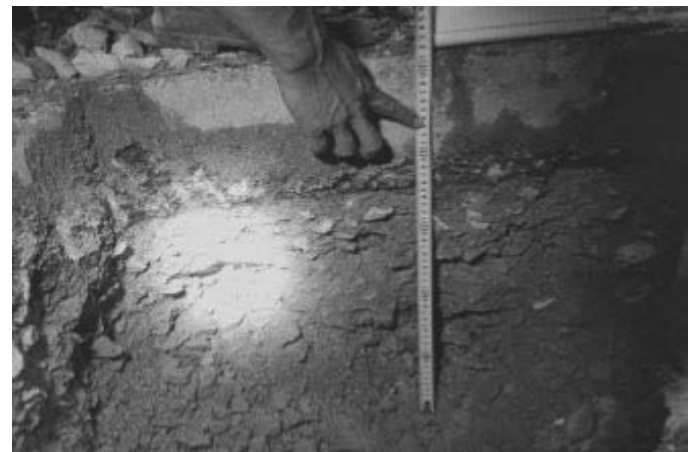
Figure 2. Excavation for exploration - evaluation of present pavement structure
