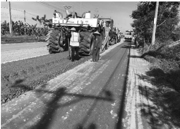
Figure 1. In the Out-of-Town route, the CIR of Rung Sac - Ho Chi Minh City is being built.
