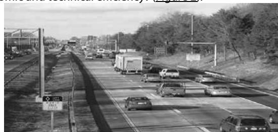
Figure 2. PPCP that has been fully constructed
