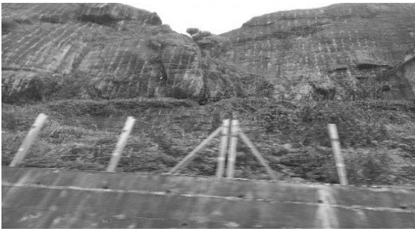
Figure 7. Hybrid protection wall - protection rock net - rock
