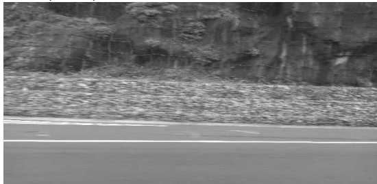
Figure 3. Gabion retaining walls
