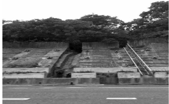
Figure 6. Rock bolt (Nailing)/anchor
