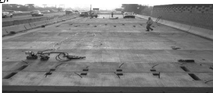
Figure 1. PPCP are being built and assembled in preparation for cable tension
