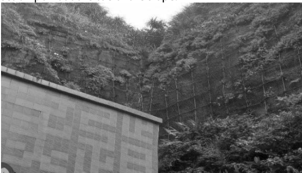
Figure 8. Hybrid barrier wall - protection rock net
