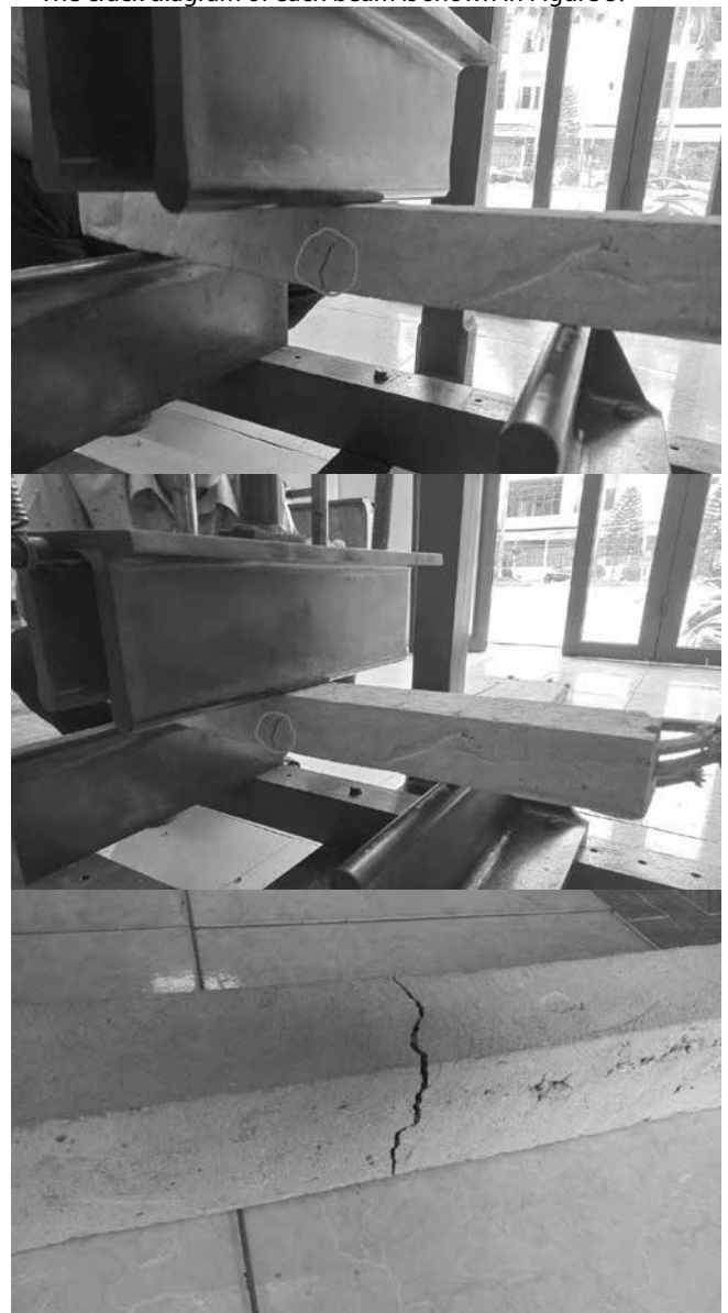
Figure 5. Crack pattern for the tested beams
