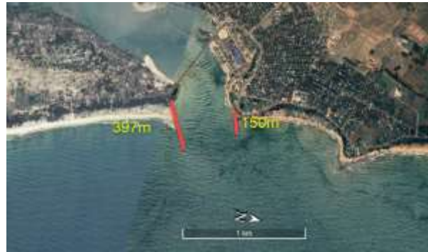
Figure 2: Jetties at north and south sides of Cua Tung estuary
