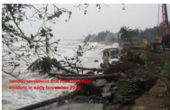
Figure 1: Incident of bank and revetment wall erosion at Cua Tung beach in 2010
