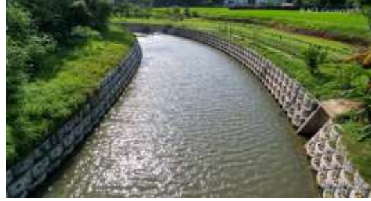
Figure 5: the applied the ACEModule™ technology for riverbank protection (a) the construction was building and (b) after the project is completed. ( https://www.geoace.com/ )
