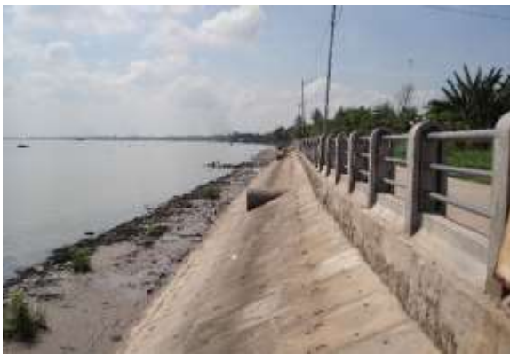
a) Concrete riverbank
