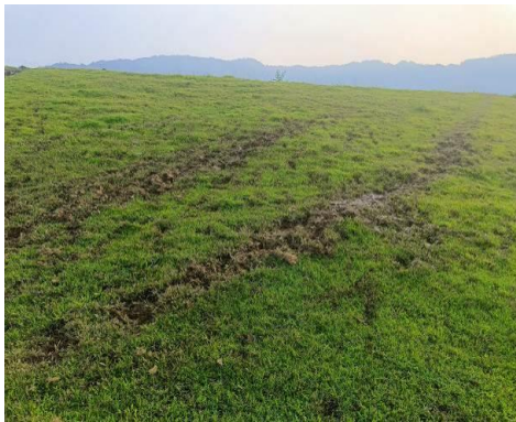
Figure 4: Seepage areas on the downstream slope of Co Dung reservoir dam
