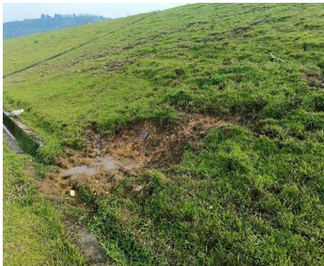
Figure 4: Seepage areas on the downstream slope of Co Dung reservoir dam
